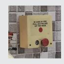
In case the kitchen personnel or someone else detects a fire before the sensor hose has reacted, he or she can trigger the activation manually. There are two manual actuation options available. The silver safety pin must be pulled, and the red strike knob must be pushed deeply and firmly. These triggers are mounted at the end or in line with the sensor hose.
